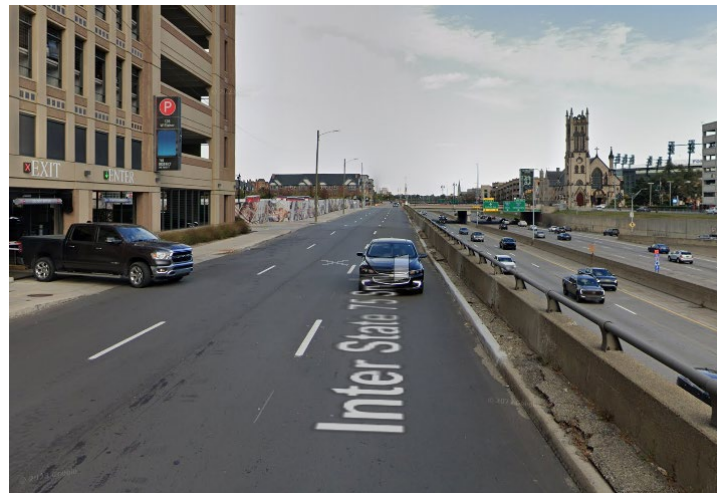
Fisher Service Drive North of I-75
