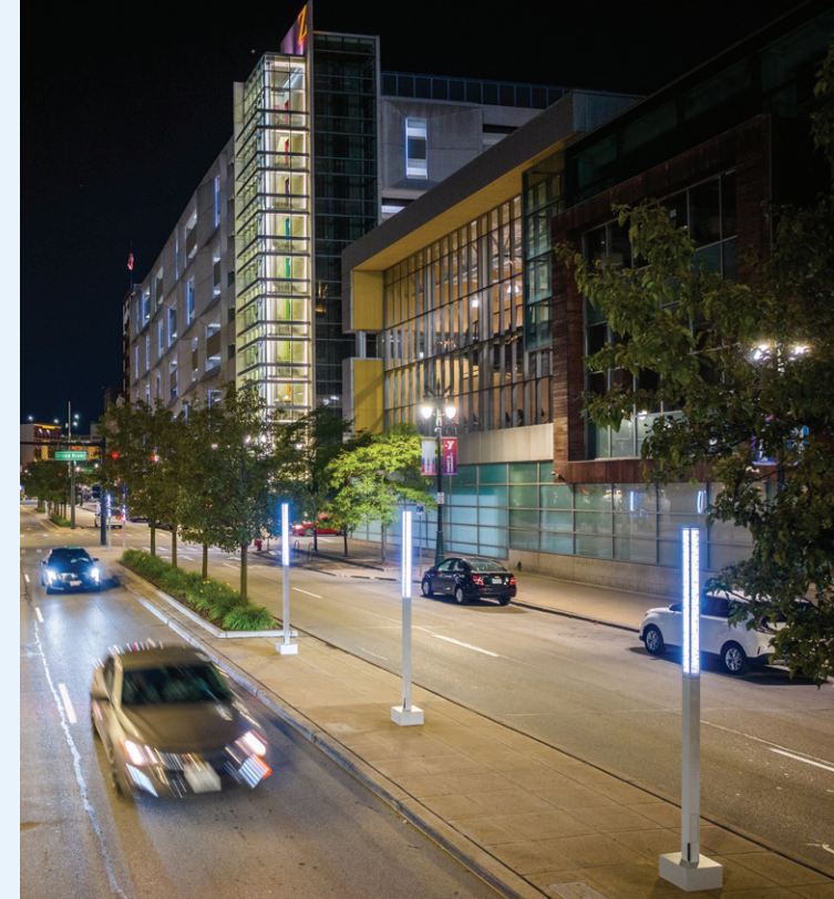
Supplemental lighting along Broadway Street
